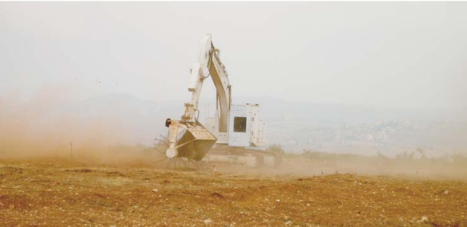
An excavator fitted with a flail in Lebanon
