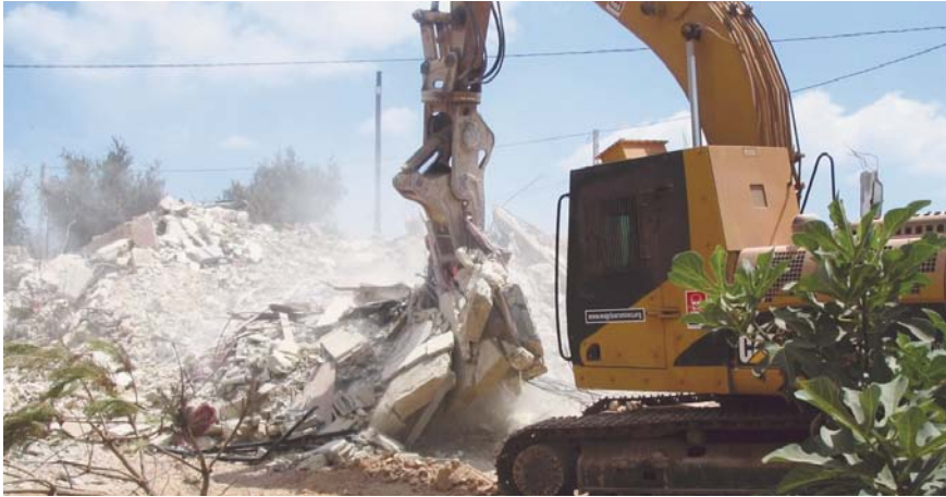
Rubble removal in Lebanon
