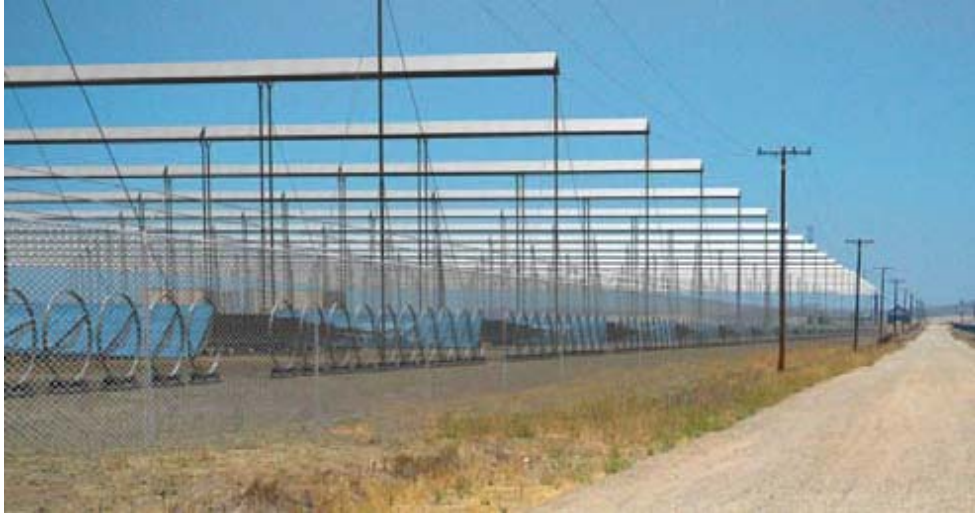
Figure 3.5 Visualisation of 177 MW e plant based on Fresnel-lens at the Carrizo Plain, CA Source: Internet Source 13.
