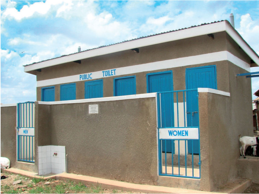
An improved sanitation facility stands unutilised by the community because they cannot afford the cost of accessing it
