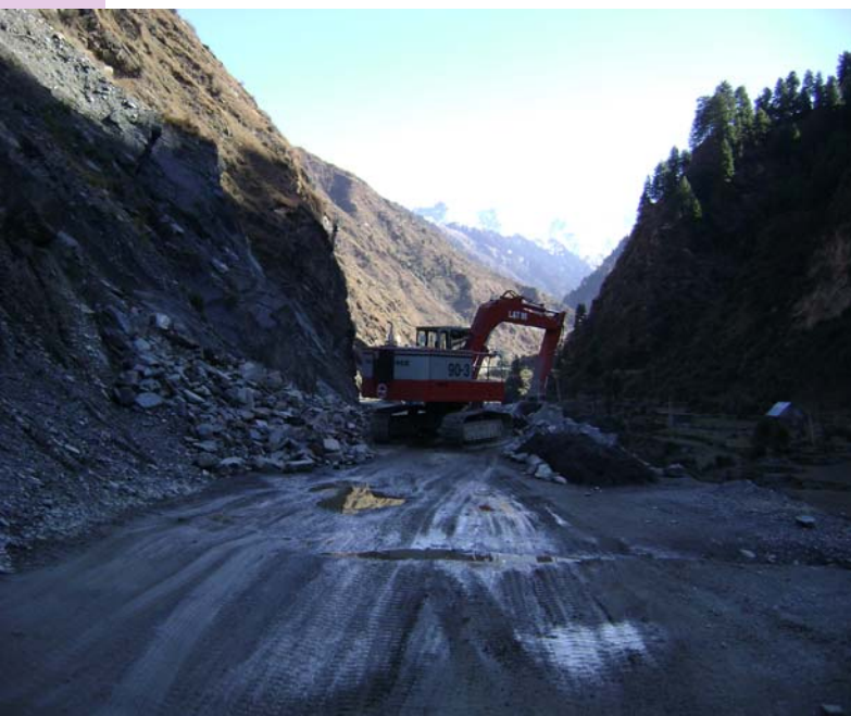
Under Reconstruction: The heritage Mughal Road across the Pir Panjal
