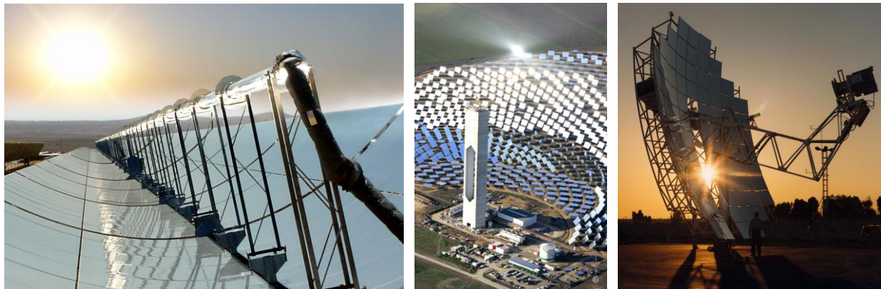
Figure 1: Parabolic trough, tower, and dish CSP technologies
