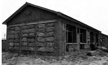
Construction of straw bale building (Photograph courtesy of ADRA)
