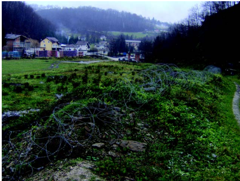
The security fence of the Kiseljak Ammunition Depot. Officers in charge said they needed more wire, as well as concrete and earth-moving equipment in order to finish the job as the security was not, in their view, adequate. Note the proximity of the nearby village.
