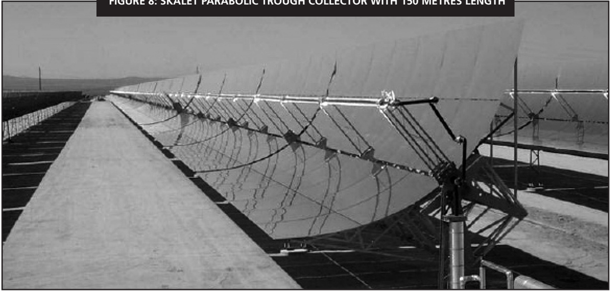
FIGURE 8: SKALET PARABOLIC TROUGH COLLECTOR WITH 150 METRES LENGTH
