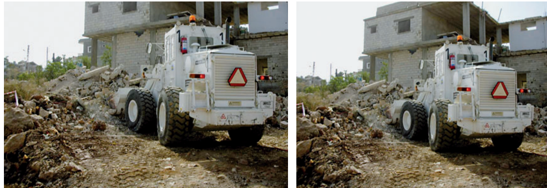
MSB Front-end loader moving rubble (Photo by Magnus Bengtsson)
