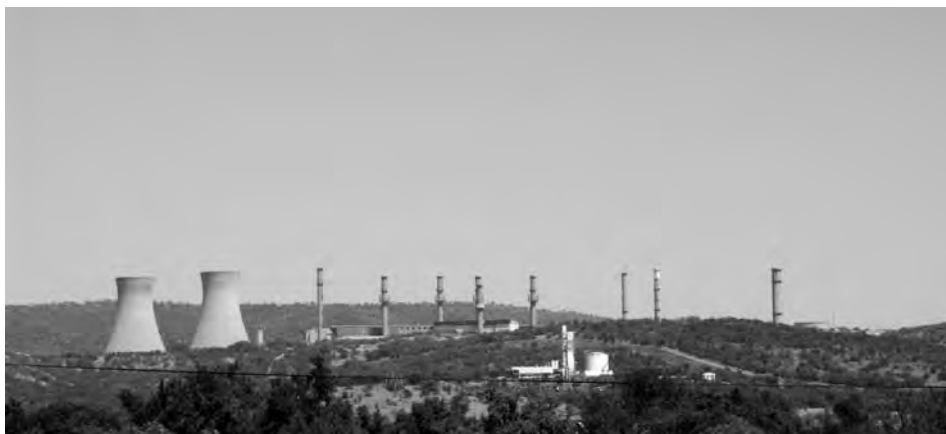
The Pelindaba Nuclear Research Facility, Pretoria, South Africa (Picture by Necsa)
