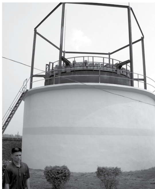
The Cang Dong biogas digester ( shui feng chi ) has a massive “floating” cap, which gets pushed up by the biogas. The cap is weighed down by cinderblocks, creating pressure sufficient to drive the gas the 2 kilometers to the village and the electricity generator. © Ben Greenhouse
