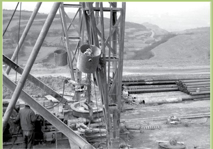
CMM Project Construction at Jincheng Mine in Shanxi Province. ©U.S. Environmental Protection Agency
