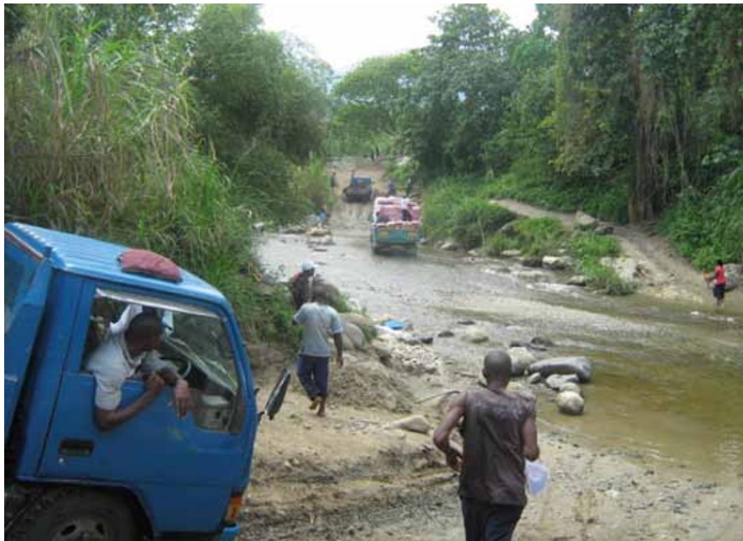
Road and bridge infrastructure damaged by heavy rains in Bundibugyo.
