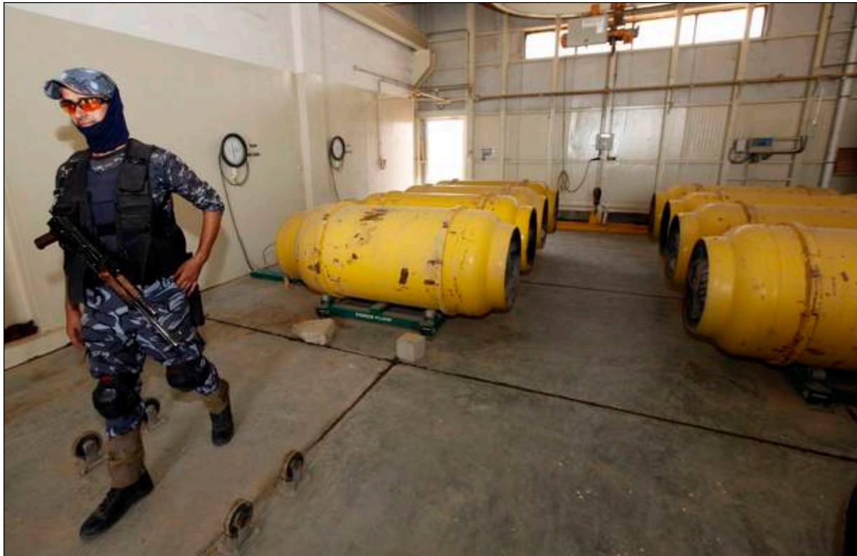
Figure 2: One-ton (840 liter) chlorine tanks at a major water treatment plant in Iraq. Almost all one-ton tanks found in Iraq are this model and are painted yellow.
