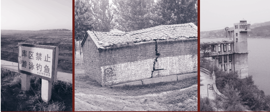
1-No Fishing or Swimming sign on the “bank” of Daning reservoir.; 2-Building in the outskirts of Beijing destroyed due to settling caused by falling water table.; 3-Guanting Reservoir now holds only a fraction of its capacity. Photo credit: Wang Jian.
