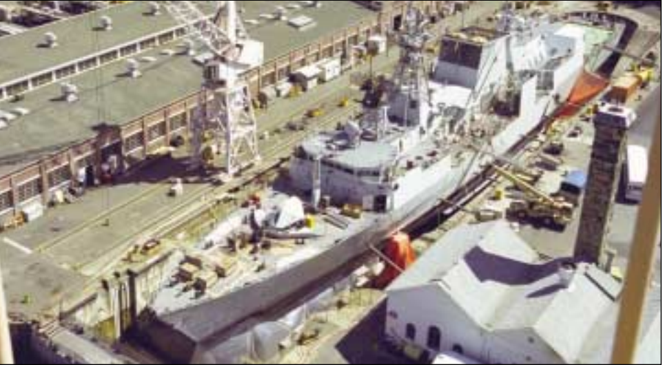
National Ship Repair Facilities — Graving Dock— HMC Dockyard, Esquimalt, BC. (CF Photo)
