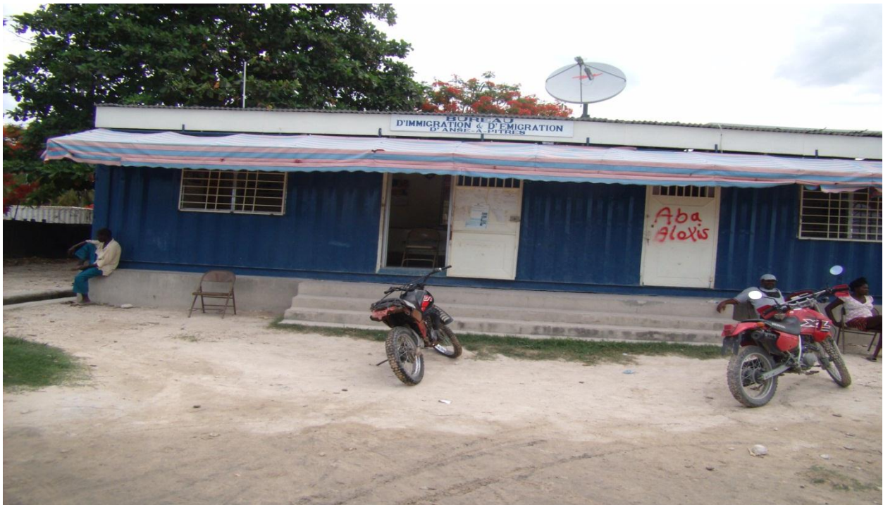
Offices of Haitian administration at the border (Immigration and Emigration) on the Haitian side. People are ashamed of these « officers » whereas at the other side, the Dominican state has provided decent offices for customs, immigration and the army battalions.
