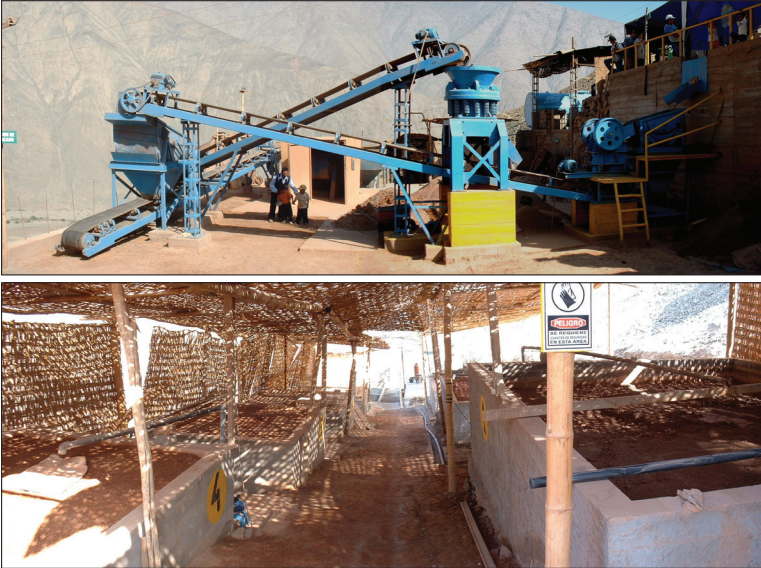
Figure 16: Initial processing plant of SOTRAMI with vat leaching section, upgradeable for later agitation leaching. Santa Filomena, Peru. (GAMA 2002)
