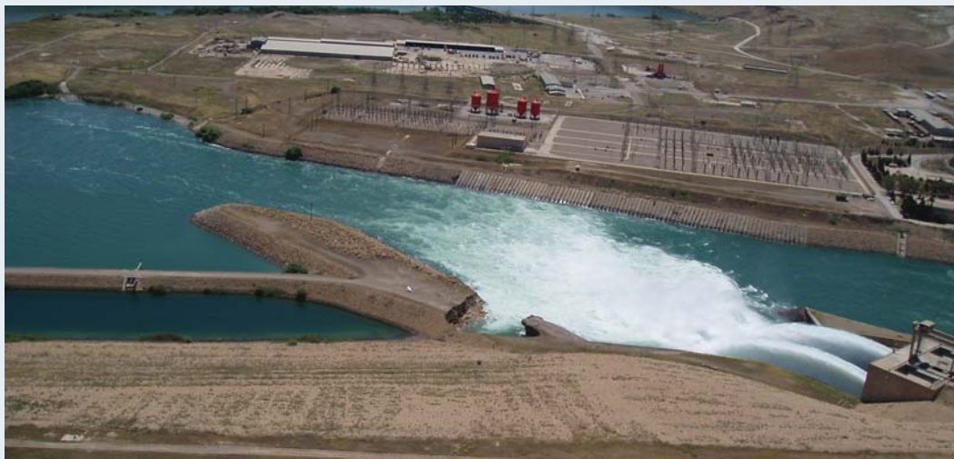
The Mosul Dam supplies drinking water, irrigation, flood control, and hydroelectric power to the surrounding region. (IRMO photo)
