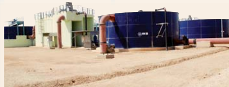
After: Completed WWTP in 2011
