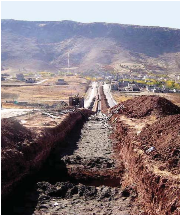
Approximately $350 million in CERP funds were spent on transportation projects, mostly for road construction.
