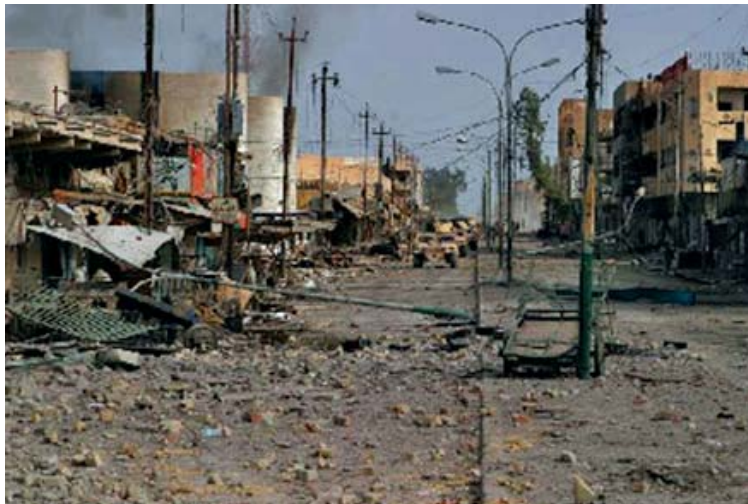
Falluja had become a lawless, chaotic place by mid-2004, with insurgents in complete control of the city, yet in June of that year the CPA awarded a $28.6 million task order calling for the completion of a new sewerage network by February 2006. (USACE photo)
