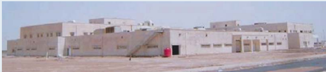
USACE expected to complete ESF-funded construction of the Missan Surgical Hospital by the end of 2012. (USACE photo)
