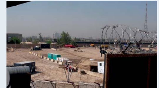
INL spent more than $100 million renovating facilities at former Forward Operating Base Shield, which was to be the main PDP basing area, before terminating construction, removing all advisors from the site, and turning the property over to the GOI.
