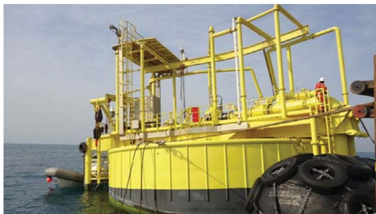
Single-point mooring station off al-Faw. (Leighton Offshore photo)
