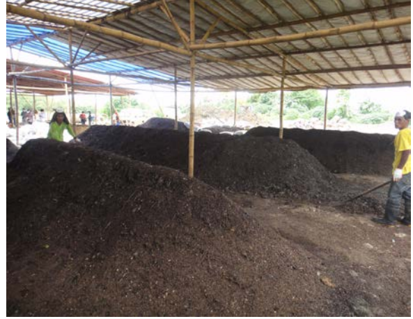
Figure 8. Central composting facility in Inayawan
