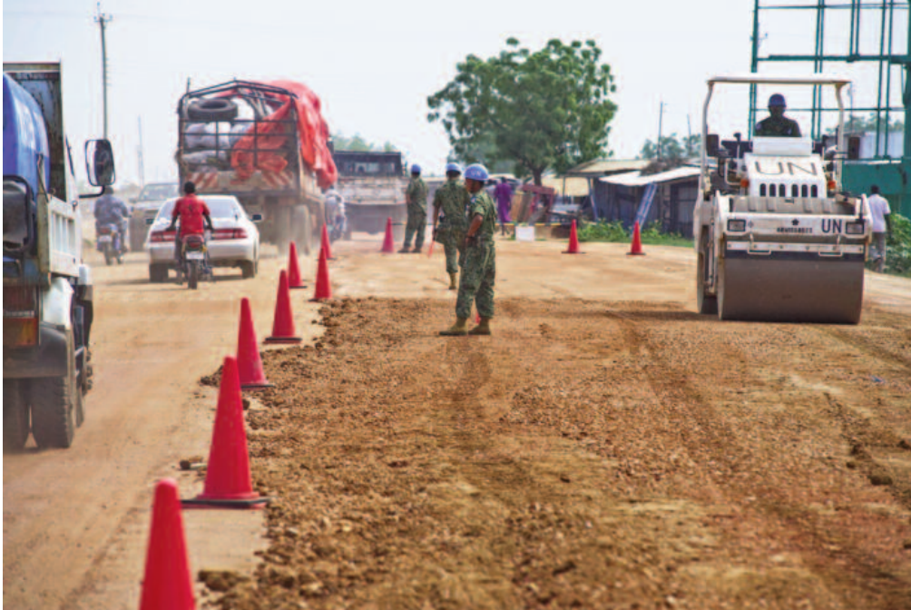
Japanese engineering peacekeepers serving with UNMISS upgrade Yei Road in Juba in August 2012. UN Photo/Staton Winter.
