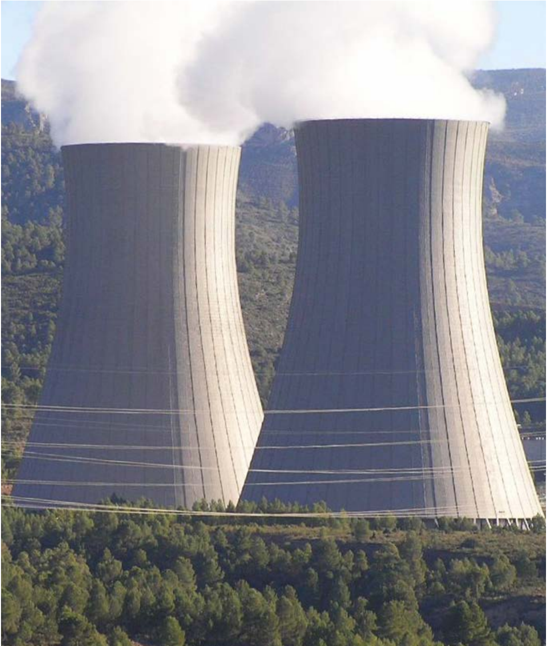
Cofrentes nuclear power plant cooling towers. Photo credit: Wikimedia Commons
