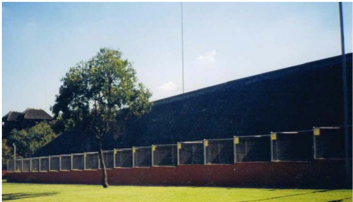
Fig. 1a. View of front kennel block.
