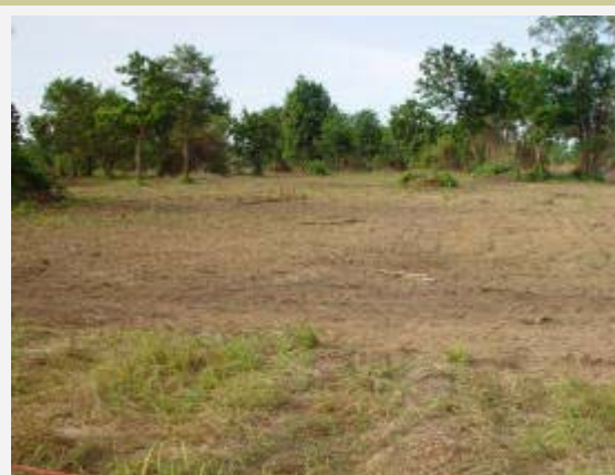
A mechanically prepared area in Thailand. Vegetation is cut and collected, hard soil loosened and the majority of metal contamination removed with the use of a powerful magnet. c/o L. Kaminski
