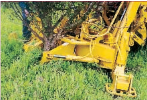
The Pearson Tree Extractor removing a tree
