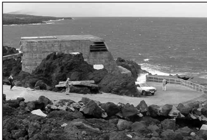
A wave-power plant on the Island of Pico in the Azores. The power rating for this plant is about 600 kW.
